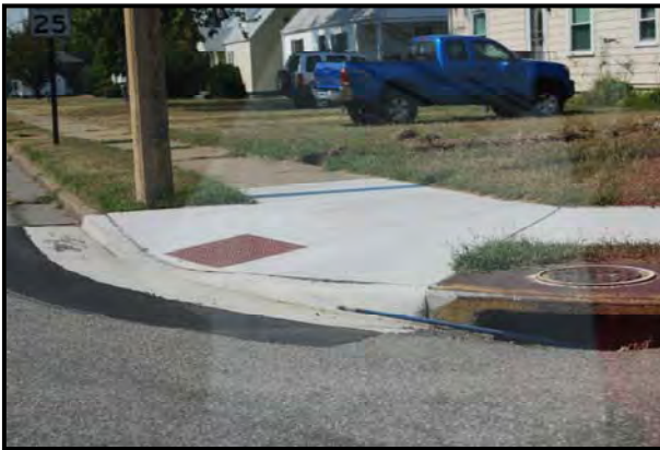
Curb is now handicap accessible
