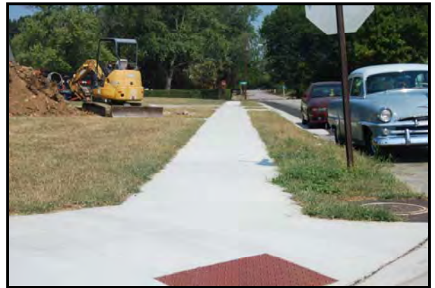
Installation of sidewalk/increase pedestrian access
