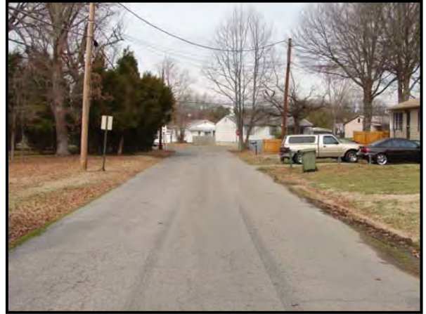
Narrow Street/ No curb and gutter
