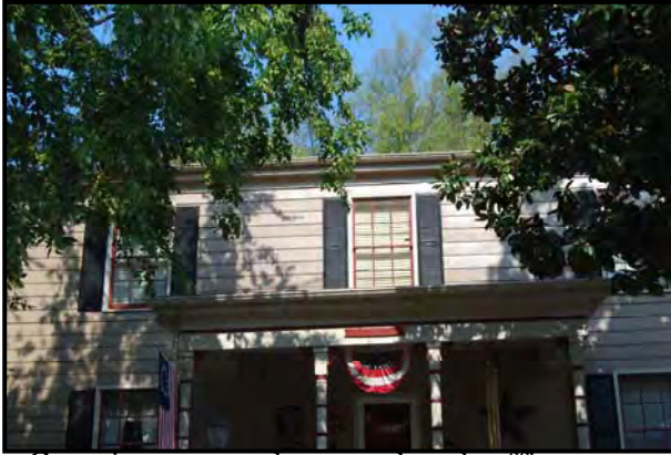
Guttering system along porch and soffits
