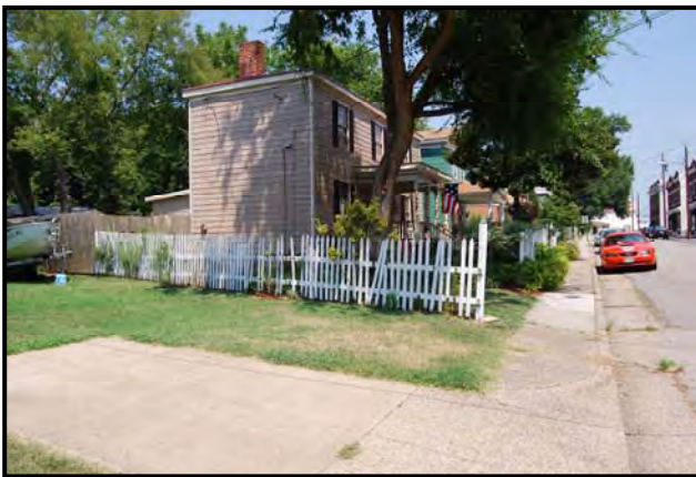
Deteriorated fence from the west home
