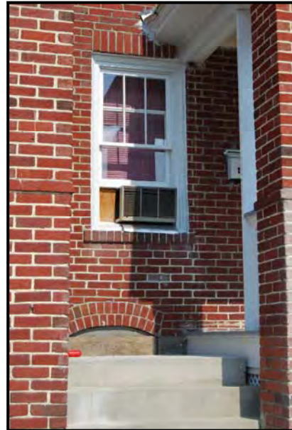
New steps that are in-line with porch floor
