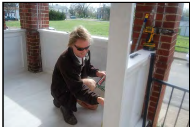
New porch flooring
