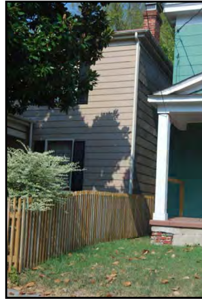
Guttering system along side of home
