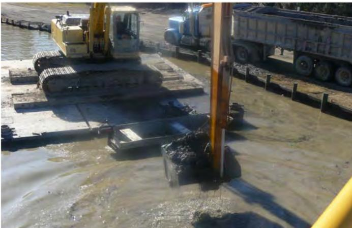
Hopewell City Marina completes dredging project with 8700 cubic yards of material removed from the marina which is made up predominately of clay, silt and sand. The last time the Hopewell City Marina was dredged was 1988. Hydraulic dredging was used around the slip areas with the material placed in bags to dewater. Other areas of the marina were dredge mechanically with over 400 truck loads taken to Port Tobacco in Charles City.
